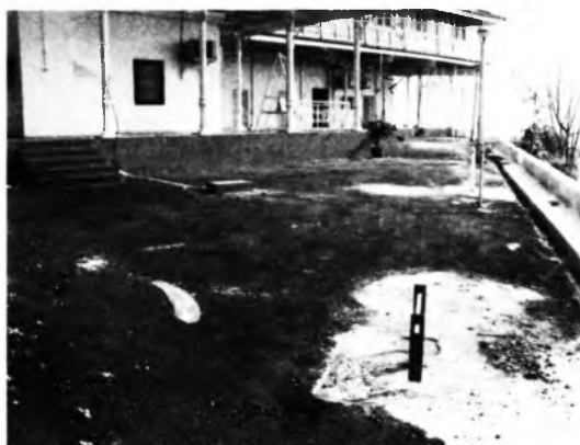
Photo : Installation of settlement gauge, inclinometer and crack recorder
