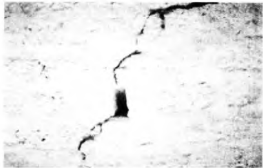
Photo : Cracks on the slope protection structures include topographic mapping on 1:200
