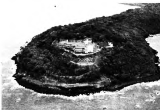
Photo : View of the Cabohill with protective measures
