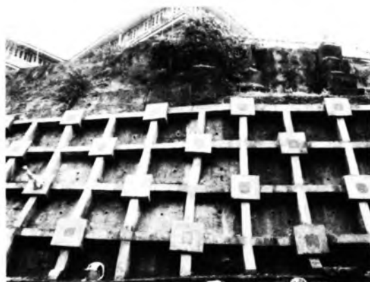
Photo : Prestressed cable anchoring at the top part of the slope
