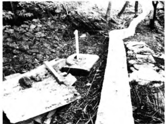
Photo : Vertical bored piles with beam caps in the midslope
