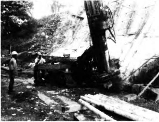
Photo : Inclined bored piles with beam caps
